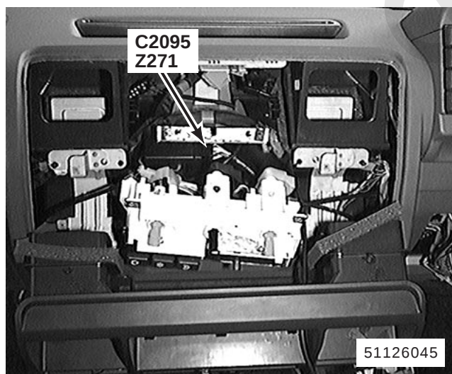
119. behind centre of fascia
